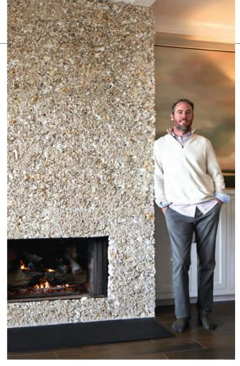
**BLAST FROM THE PAST** Tabby is a type of concrete made by burning oyster shells to create lime, then mixing it with water, sand, ash and broken oyster shells. With a few modifications, Giltner has created the same process and look for exterior and interior applications and wall finishes.
